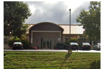
ABH's New Building West Nyack, NY
